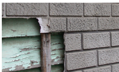
External cladding containing asbestos
