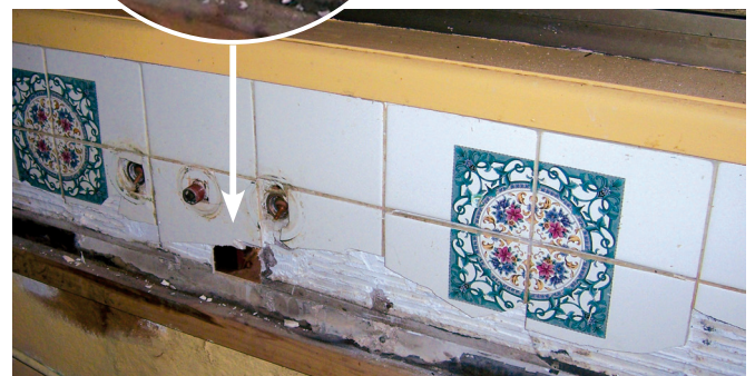
Ceramic tiles on asbestos sheeting
