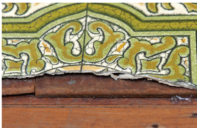
Asbestos backed vinyl sheet flooring
