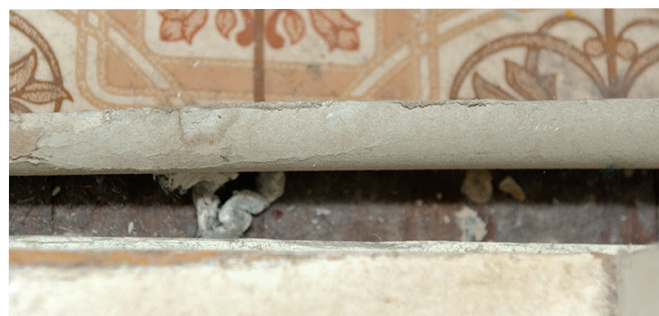
Asbestos backed vinyl sheet flooring
