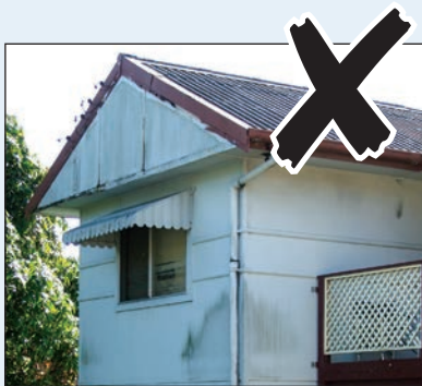
Asbestos wall sheeting
