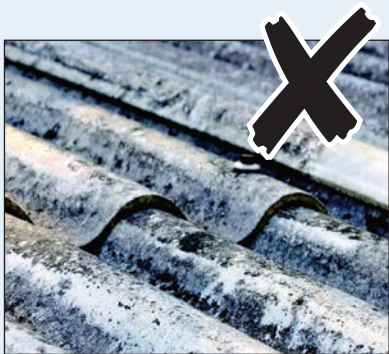
Super six asbestos roof
