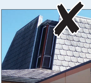
Shingle asbestos roof
