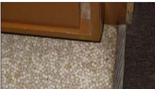
Figure 2 – Terrazzo type asbestos backed vinyl sheet flooring.
