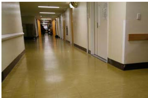
Figure 3 – Asbestos vinyl tiles © WorkSafe Victoria
