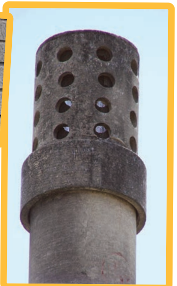
Vent pipe cap and socket fitted over a vent pipe
