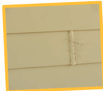
Hardi plank wall sheeting
