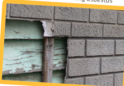
External cladding containing asbestos
