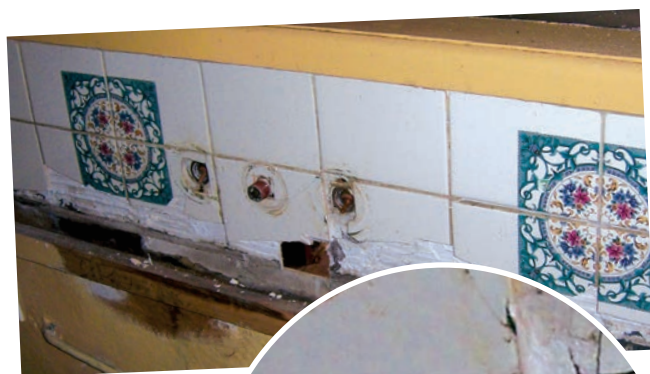
Ceramic tiles on asbestos sheeting
