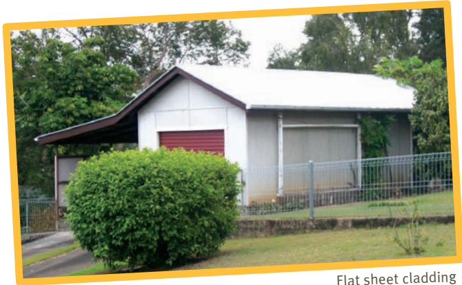
Flat sheet cladding
