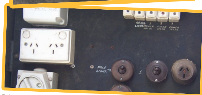
Zelemite backing board to an external switchboard
