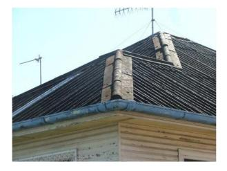
Cleaning a fibro roof with a high pressure water blaster is illegal as it can destroy the roof surface, cause cement debris and asbestos to spray into the air, and result in widespread contamination.
