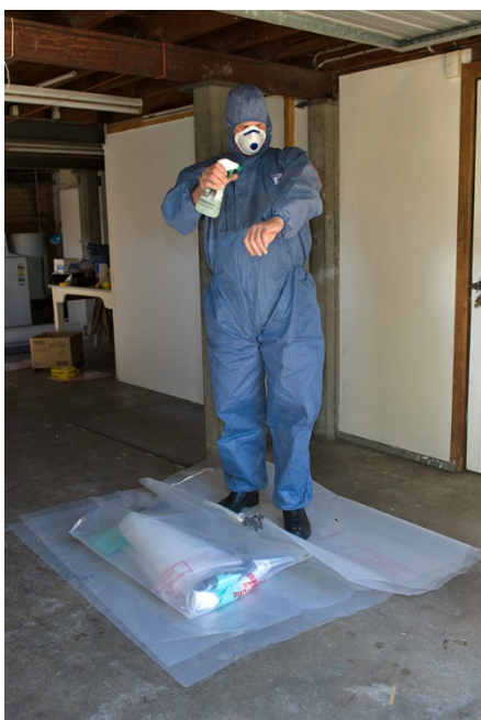
Step 1: Standing on a plastic sheet (a decontamination facility), use an atomiser bottle of water to wet the coveralls.
