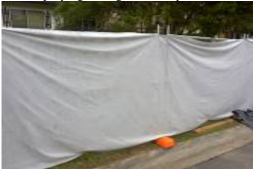
Dust barriers on boundaries of the demolition area
