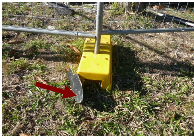
Photo 8: delaminated thin pieces of ACM should be shovelled up along with soil immediately below
