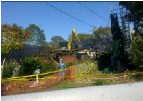
Water spraying during machinery demolition
