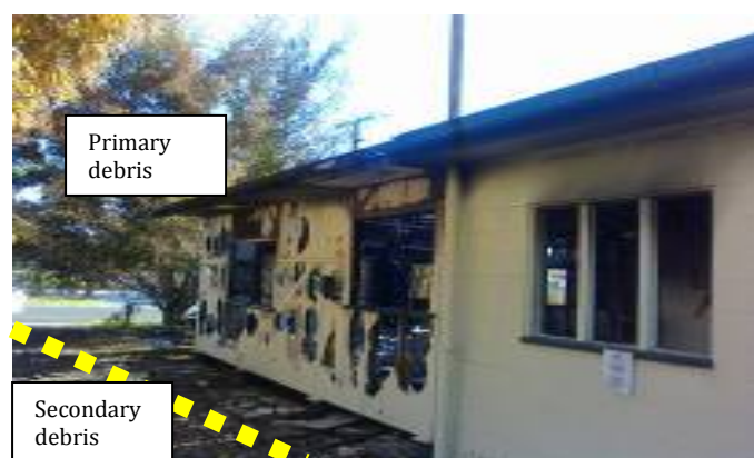
Photo 2: This single story fibro clad house was extensively damaged by fire. Confirmed asbestos containing material, from the roof, soffits, external and internal walls was found both internal to the structure and in a radius of approximately 20 metres from the structure.
