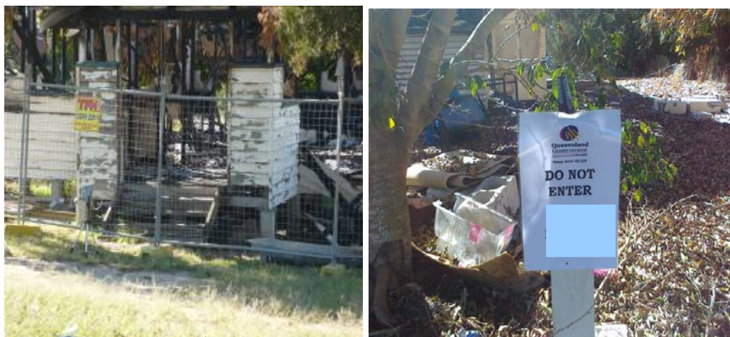
Photos 3 and 4: Examples of barriers and signage that may be required if there is a need to prevent people from entering the fire damaged property
