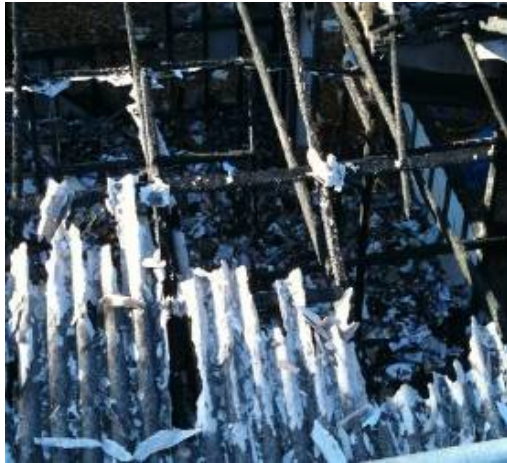
Photo 1: The high temperature of the fire has caused a spalling effect to the roof sheeting
