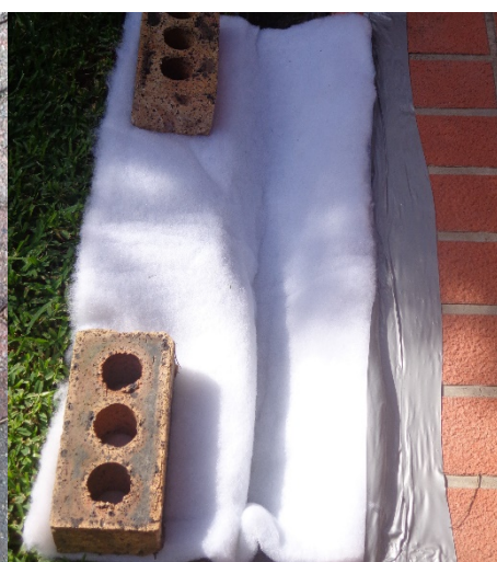
Photo 13: Filter medium in a channel in place in readiness to capture residue and filter out the water.
