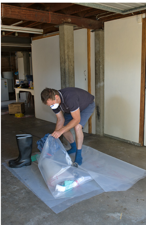
Step 4: Place the coveralls and wipes in an approved waste bag.
