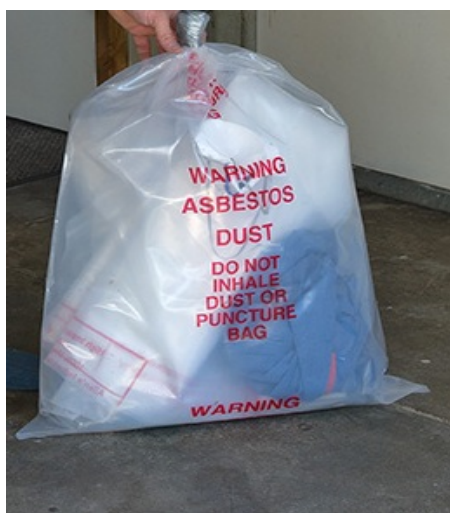
Photo 14: ACM debris correctly sealed in an approved bag.
