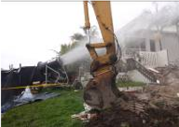
Water mist spraying during machinery demolition
