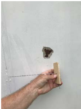
Photos 2 and 3: Coat hanger wire inserted through the patch, note right angle of the wire.
