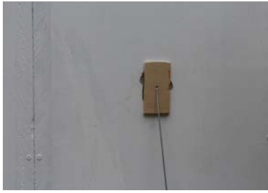
Photo 5: Pulling the wire tight and bending the wire at right angles over the timber.
