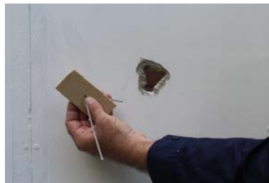
Photos 2 and 3: Coat hanger wire inserted through the patch, note right angle of the wire.
